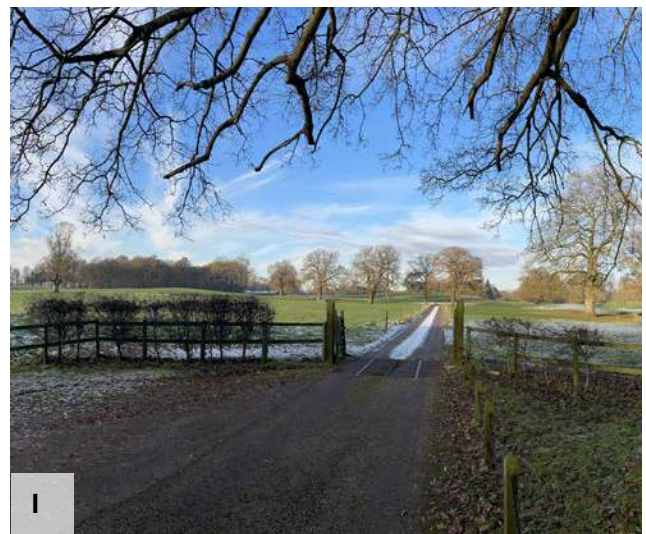
View I. View towards Birtles Hall from Birtles Lane. The landscape rises gently up towards the Hall. The estate grounds in this view represent the wider parkland setting of the house.
