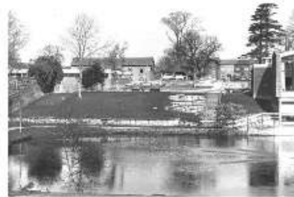
Y. Black and white photograph of water garden, looking north, c.1963
