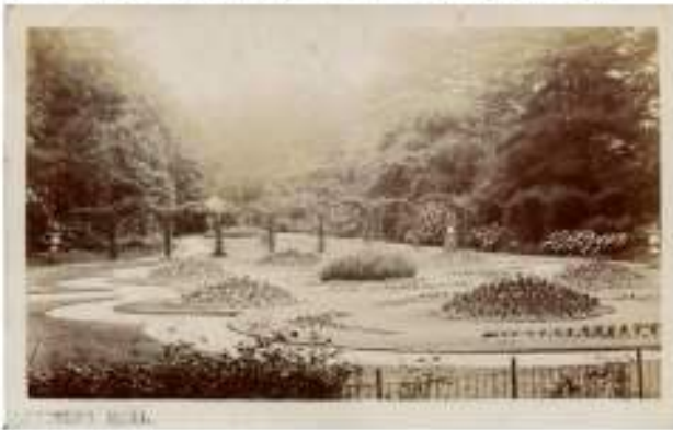
6. Postcard of Birtles Hall postmarked 12 th January 1908. This photograph appears to show the northern garden separated from the original garden by railings. It is formally laid out with circular mounded beds for bedding, ornamented with urns and crossed by a line of arches with climbing plants. To the rear is a summerhouse or shelter, possibly circular and with a thatched roof, the small building shown on the 1910 Ordnance Survey.
