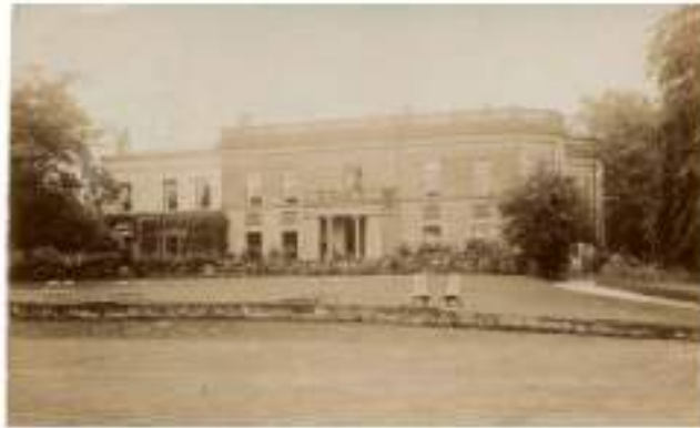
10. Postcard of Birles Hall postmarked 4th July 1915 (signed Gilbert) of the south elevation with the west wing that was demolished in 1937. It shows planting along the balustrade, a low stone retaining wall marking the line of a possible former ha ha, and the former tennis court now laid out for croquet.
